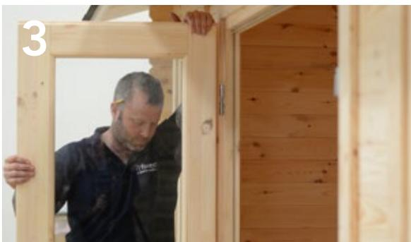
Carefully lift the door back onto the door frame hinge and check the adjustment. If further adjustment is required, lift the door back off the hinges and repeat the process as required.
