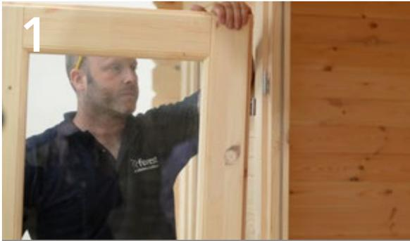
Start by lifting the door off the hinge.
