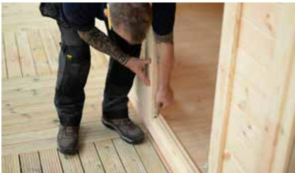
When adjusting the doors, line the internal locking bolts up with the bolt holes located in the door frame. This will act as a guide on how far each door should be adjusted. In cases of extreme movement, the bolt holes may have to be relocated by drilling a new receiver hole, unscrewing the metal bolt hole cap, and re-screwing it over the newly drilled hole.
