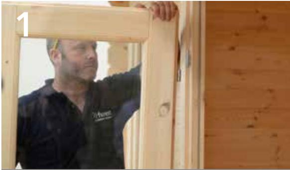
1 Start by lifting the door off the hinge.
