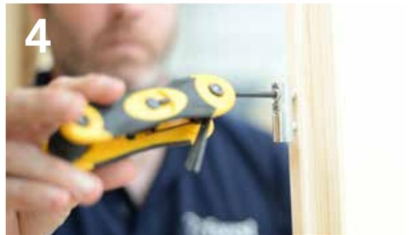
4 Using an Allen Key, turn the adjustment bolt anti-clockwise to push the door closer to the adjacent door, or turn it clockwise to pull the door back towards the door frame. Repeat with the bottom hinge as necessary.
