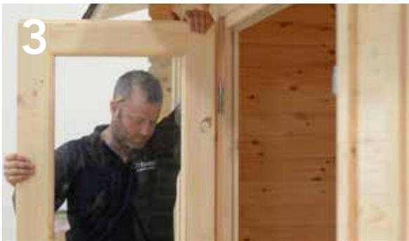
3 Carefully lift the door back onto the door frame hinge and check the adjustment. If further adjustment is required, lift the door back off the hinges and repeat the process as required.
