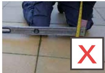
Slab base has a water run-off allowance making the base run out of level by more than 10mm.
