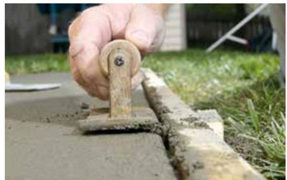
Ensure the concrete is completely dry before removing the shuttering to prevent the sides of the base crumbling away.
