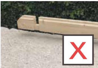
Concrete base running out of level by more than 10mm.
