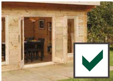
Slab base perfectly level across both the width and depth.
